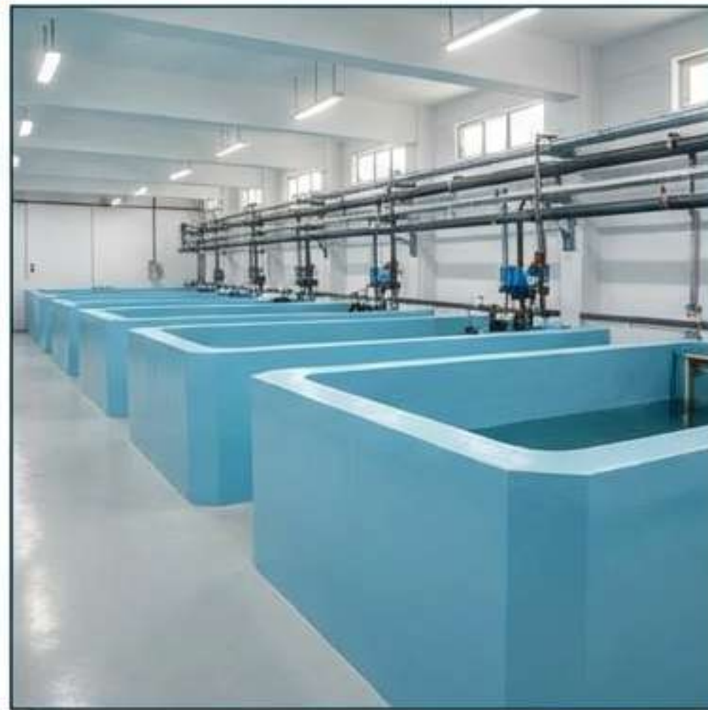
Hatchery Infrastructure & Epoxy Painting
